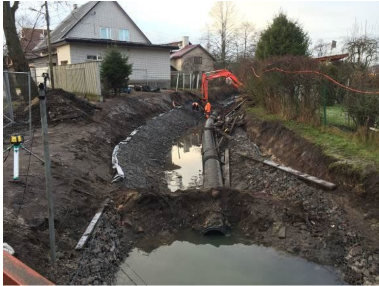
Fig. 7. Temporary draiage of the stream using barriers and drainage pipes.
