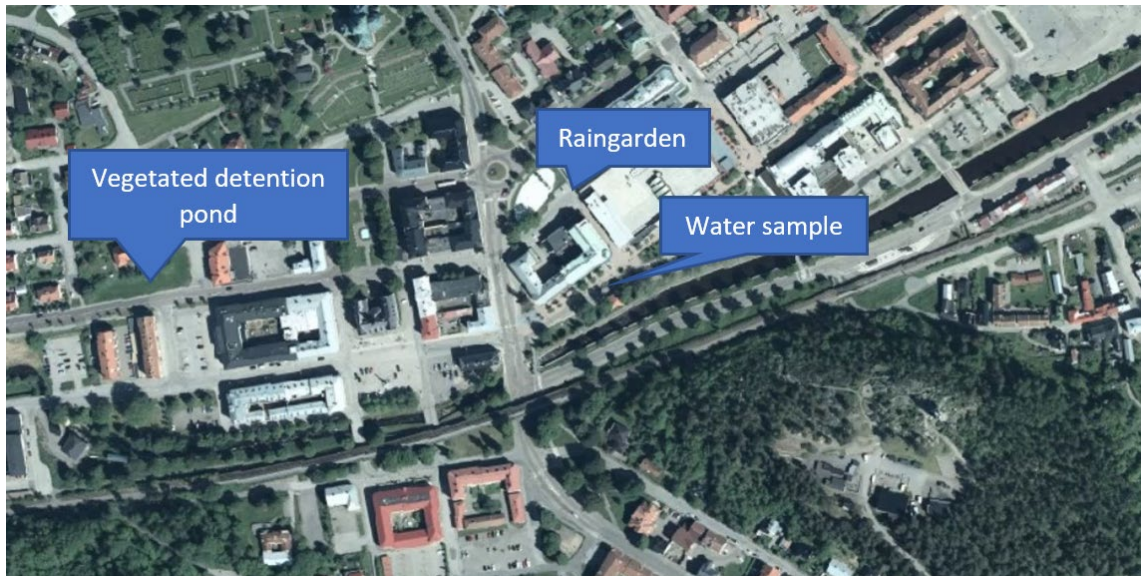
Fig. 51. Construction sites for the raingarden and vegetated detention pond. Place for stormwater sampling.
