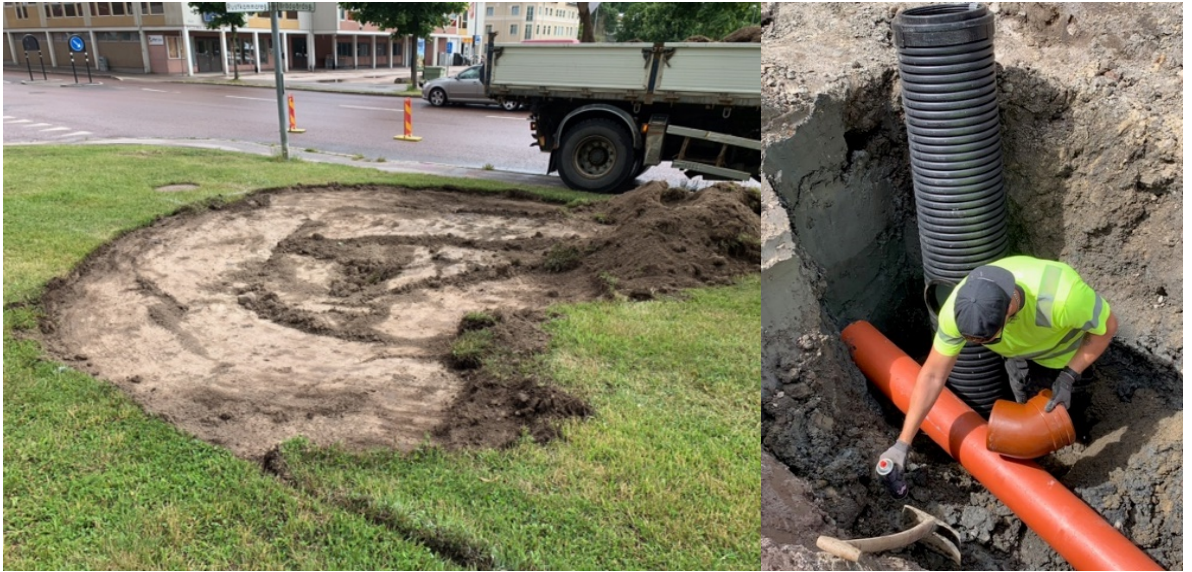
Fig. 23. Digging for the vegetated detention pond and installation of pipes.
