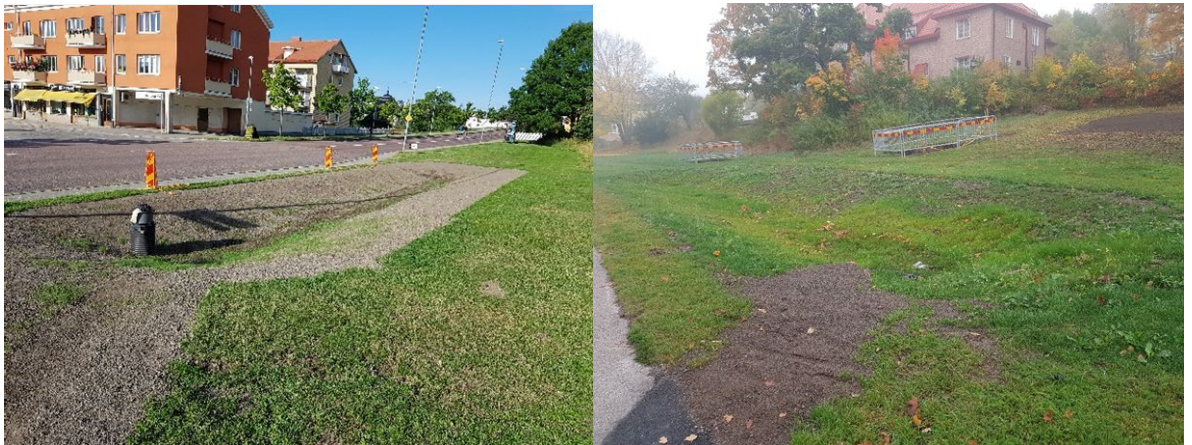
Fig. 24. Finished detention pond at Brädgårdsgatan.
