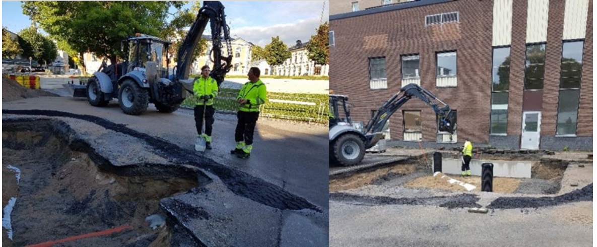
Fig. 25. Excavating the raingarden and installing pipes.
