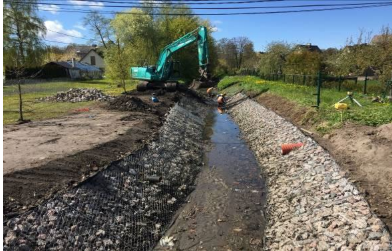
Fig. 9: Placement of the gabions for bank enforcement.
