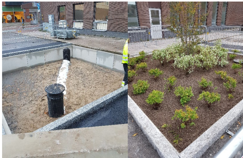
Fig. 30. Left) bed and overflow of the raingarden. Right) finished rain garden.
